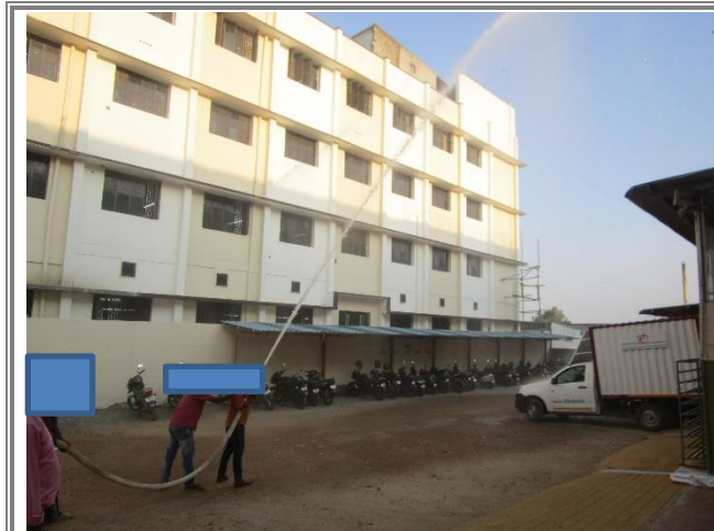
Fire hydrant tested
